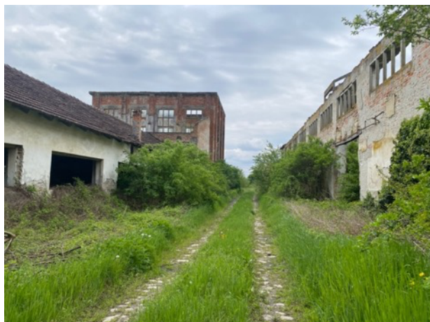
Abandoned and damaged facilities in Baranja.
